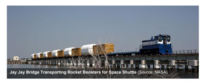
A critical component of the system is the Jay Jay Bridge (over the Indian River), which was refurbished between 2005 and 2009.<sup>185</sup> The bridge continues to be capable of handling 12-foot wide and 150-ton rocket component.<sup>186</sup>
